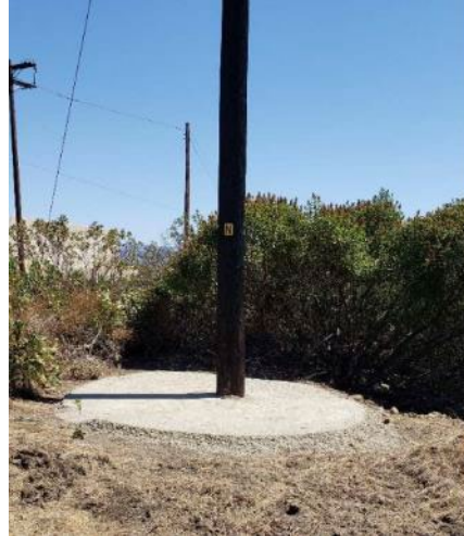
Figure 19. A minimum of 10 feet of clearance should be maintained around utility equipment.
