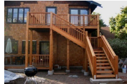
Figure 20: Deck with Single Set of Stairs
