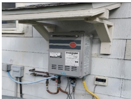
Figure 63: Wall-mounted Tankless Water Heater
