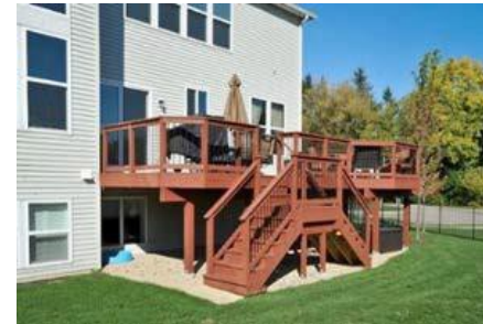
Figure 21: Deck with Double Staircase
